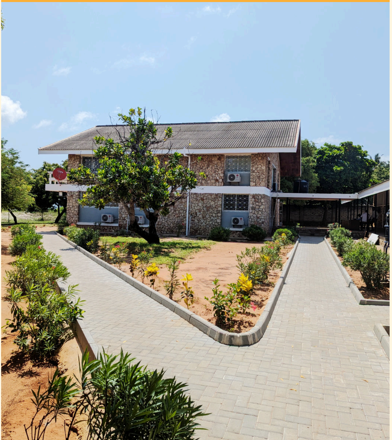
Renovated walkways at Kunduchi Campus. ©Rashidi Bilali
